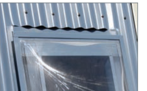
Clear (on corrugated roof profile)
